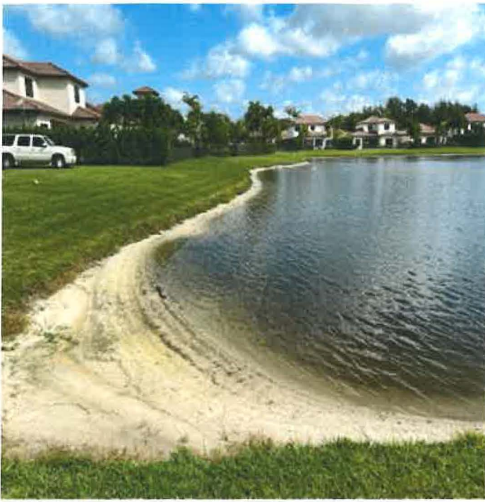
Photo 12: Lake 3 erosion by headwall
