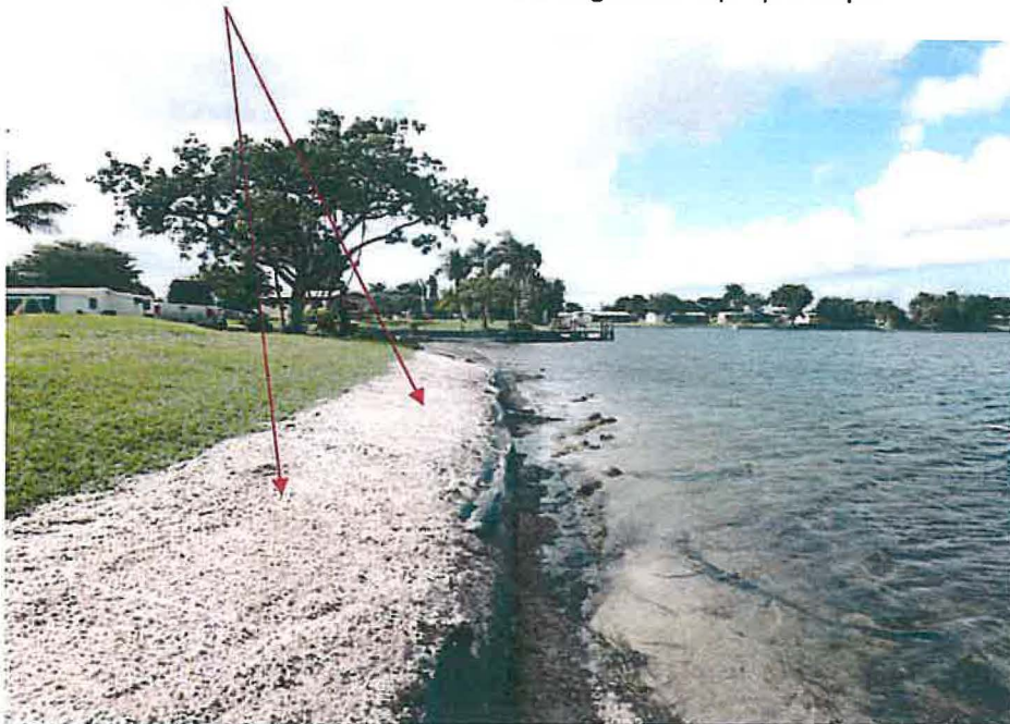
Sand installed over Geo-Tubes and graded to proper slope
