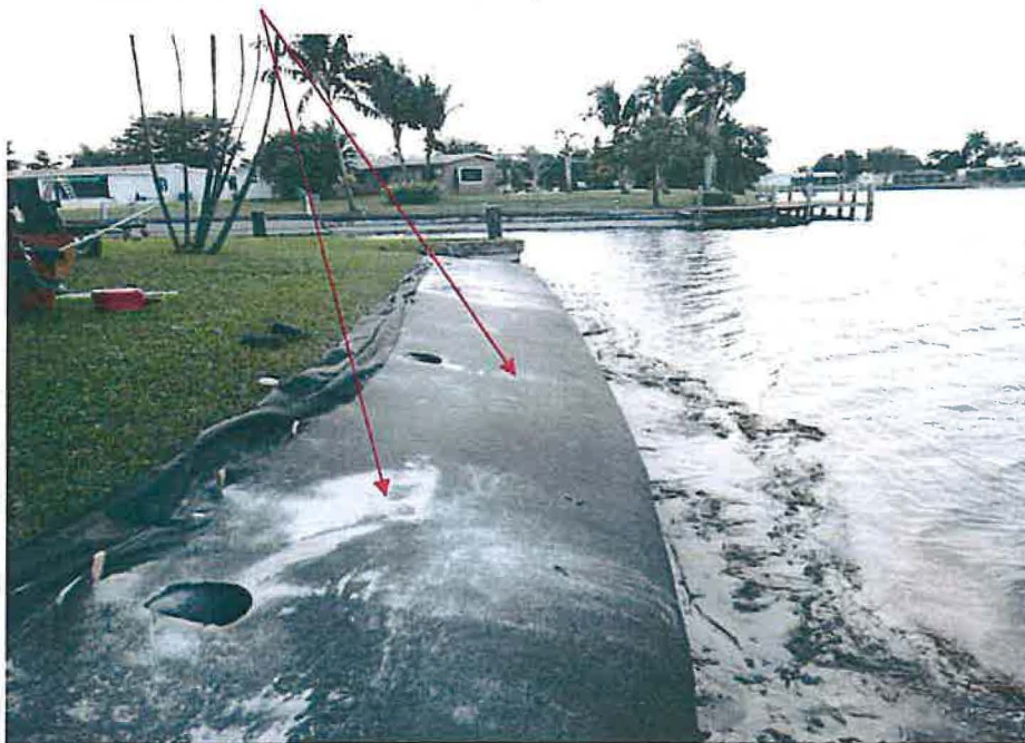
Main Geo-Tube installed and pumped with sand from lake bottom
