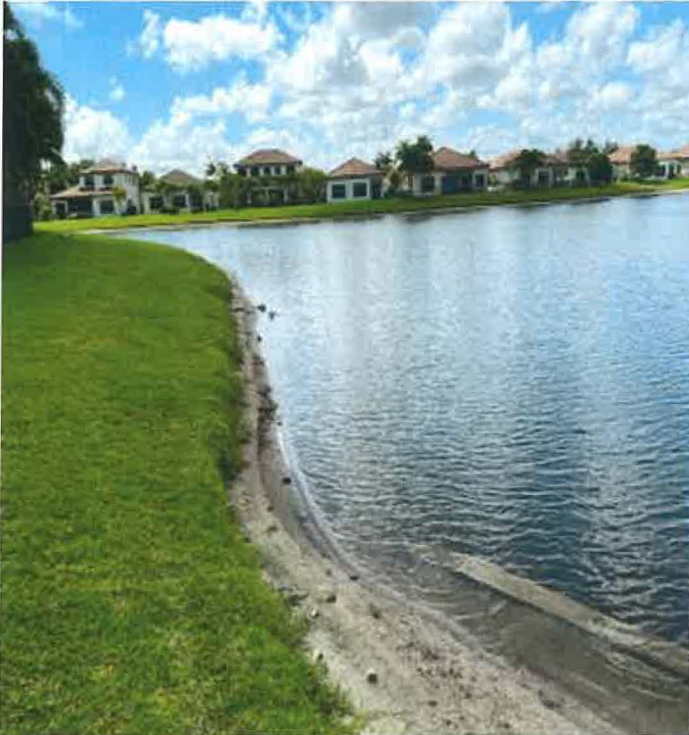
Photo 10: Lake 3 NW side erosion with 1-2' drop off
