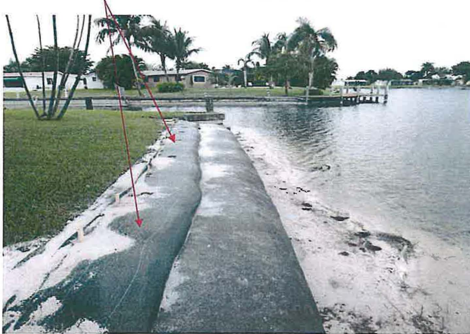
Backfill Geo-Tube installed and pumped with sand from lake bottom
