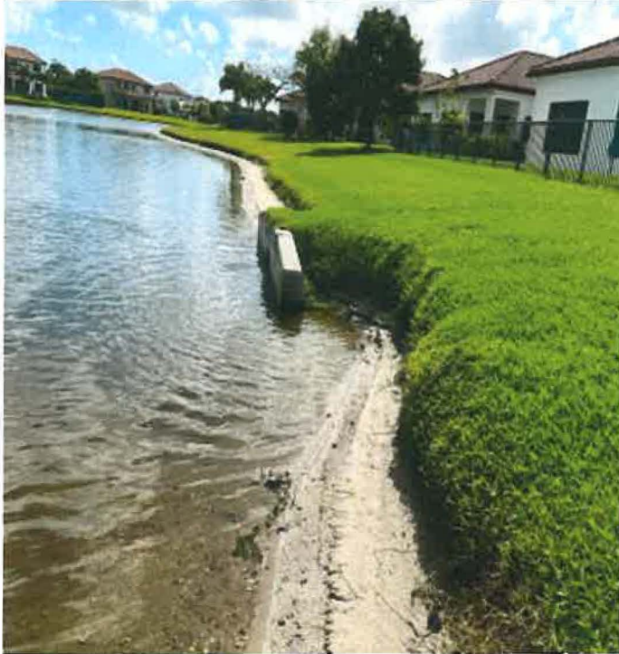
Photo 12: Lake 3 erosion by headwall
