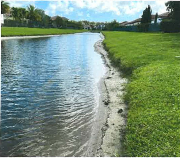
Photo 9: Lake 3 south side erosion with 1-2' drop off
